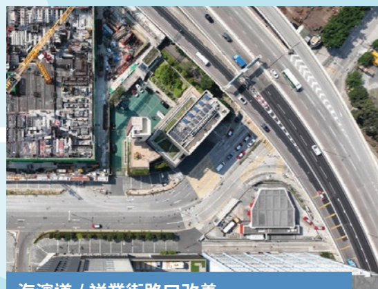
海濱道 / 祥業街路口改善 Layout improvement at junction of Hoi Bun Road and Cheung Yip Street
