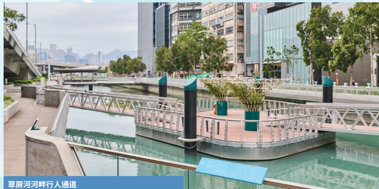
連接新急症醫院的園景美化高架行人道 Landscaped elevated walkway to the New Acute Hospital
