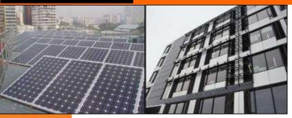
Building Roof and Facade Integrated Solar Panel
