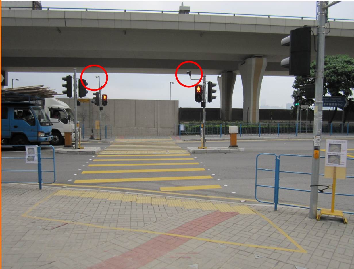
Trial pedestrian video detector at the junction of Lai Yip Street and Hoi Bun Road
